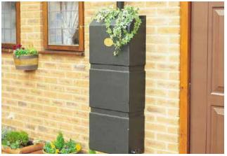
**Figure 82:** Example of a gravity fed rainwater system for flushing a downstairs toilet or for irrigation, elsewhere in the UK.
